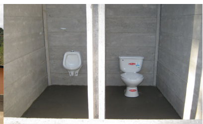
View from inside
